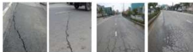
Fig. 1. Example of road crack
